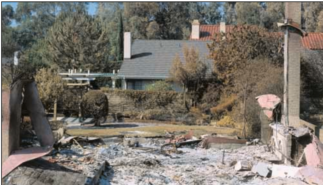
Some houses burned to the ground while other adjacent homes with metal roofing stood unscathed.
